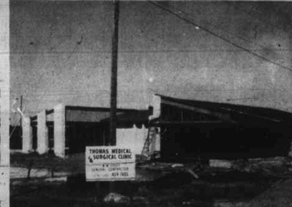
Work is well underway on a beautiful new Thomas Medical and Surgical Clinic on a site on Austin Road near the Heritage House and the Community Hospital. The clinic is a project of Dr. and Mrs. Raymond R. Thomas and will feature the latest innovations for patient and emergency services. Completion of the structure is expected by August 15th. M. M. Casey of Austin is contractor and Jim Faulk and Associates of Austin are architects.
