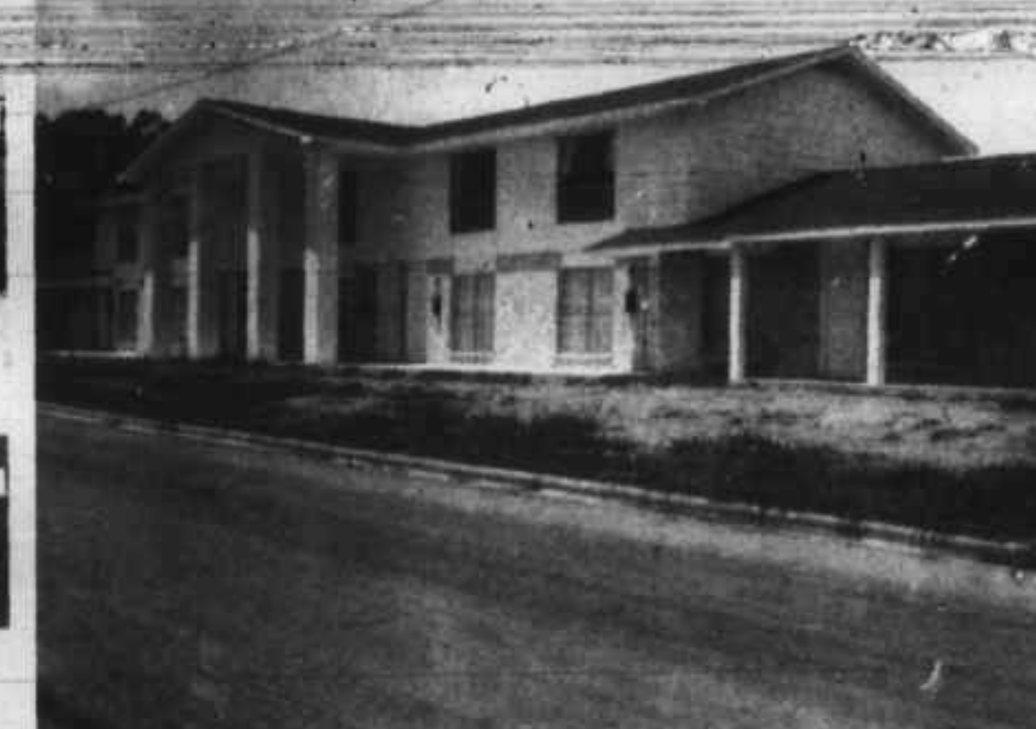
Work has just been completed on the attractive new 10-unit Eagle Lake Apartments project on Church Street in Eagle Lake. The new apartments will provide badly needed housing for this community and features ten two bedroom facilities. Owners of the project are Willard W. Shurt of Eagle Lake and Reagan Heile of Houston. Architect was Emil Zapalag Jr., of Pasadena and contractor was Fred Pelts of Columbus. The apartment is now accepting applications for occupancy.
